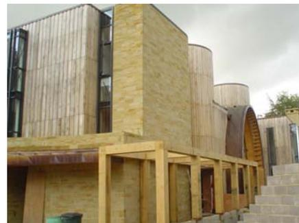
Part of the external walls have been vertically clad in timber, with selected 1–2 grade European Oak, which is FSC certificated. The timber has been fixed and allowed to start weathering naturally, using stainless fixing with the drill holes being greater than the shank to allow for movement throughout the seasons.
